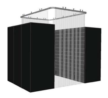
Soft wall containment can be a lower cost solution for isolating the air in hot and cold aisles.
