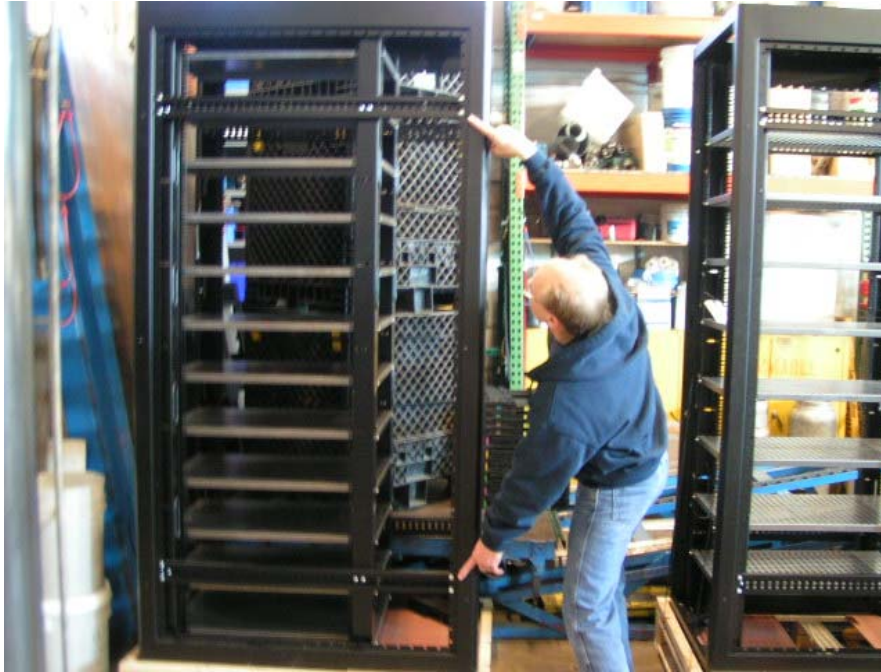
Photo 11: Location of distortion of the side rails.
